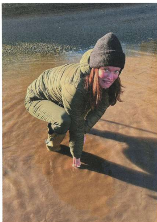
A blocked drain sending filth into a natural water-course – a not-uncommon issue
